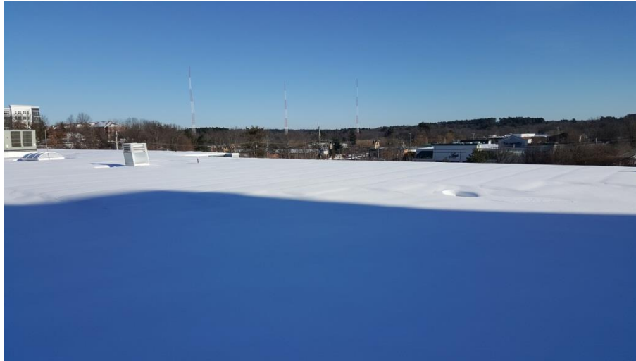
Picture 2 – Blanketed Solar Array
